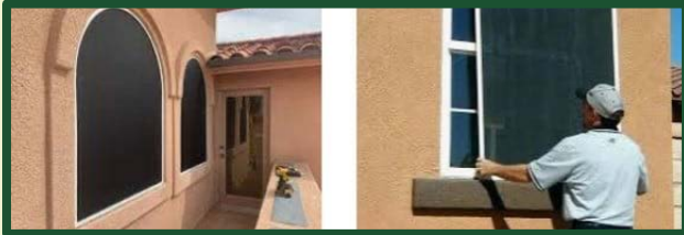
Solar screen installation
