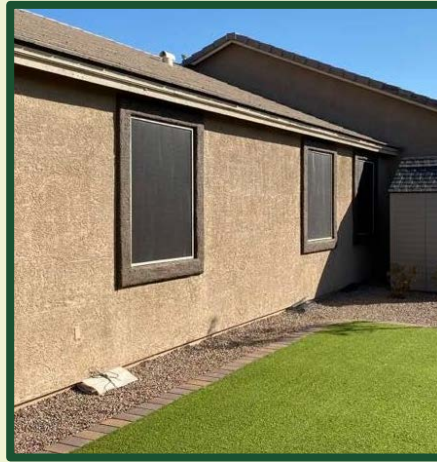
Installed solar screens
